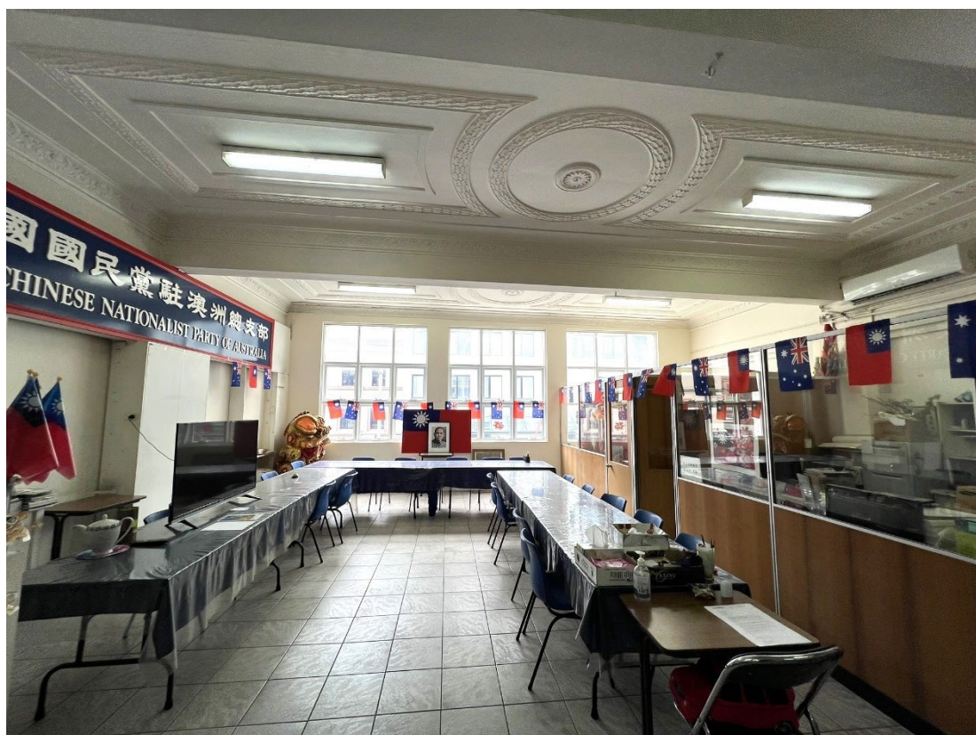
Figure 15 First floor office with plaster ceiling.
